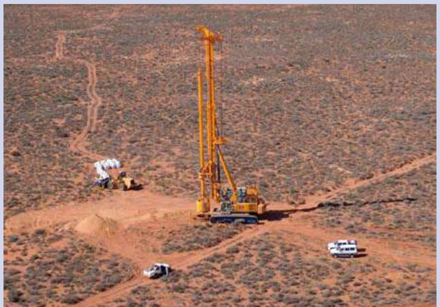
Drilling rig of Bauer Maschinen
